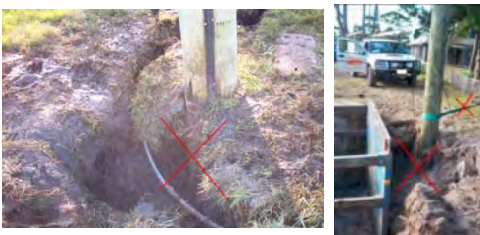
Above: Poles with become unstable if undermined
